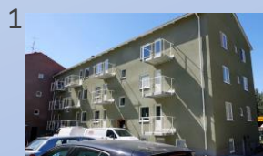
1 Kv Skidstaven, 232 st, 2017
